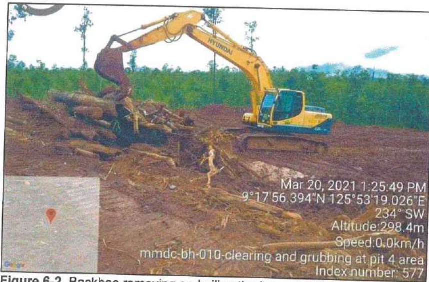
Figure 6-2. Backhoe removing and piling the logs after tree cutting activity.
