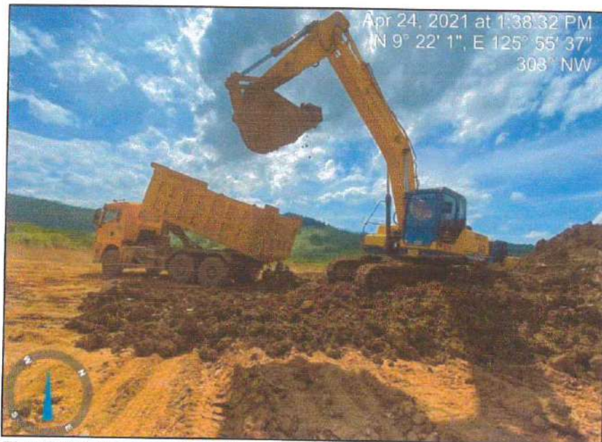
Figure 6-5. Saprolite stockpiling at MMDC Stockyards in Bon-ot, Carrascal.
