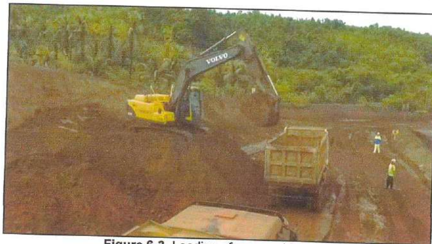
Figure 6-3. Loading of removed topsoil.
